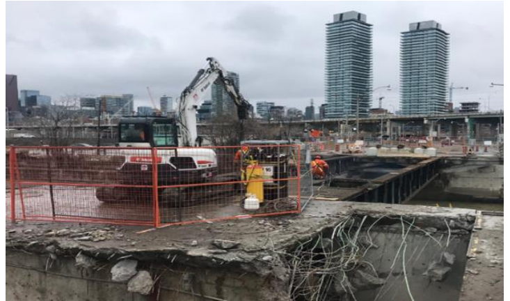
Figure 2 Old Cherry Bridge Demo - Removal of Bridge Deck
