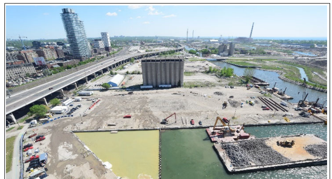
Figure 4 Parliament Lake Fill construction progress
