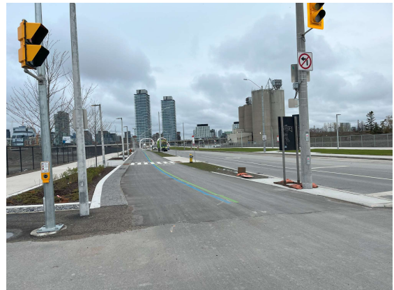
Cherry St. North – Road open and bridge in service;
