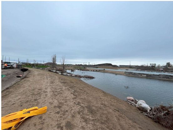
River Valley – Planting in progress;
