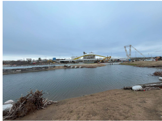
West Plug – Carp gates settlement monitoring in progress;
