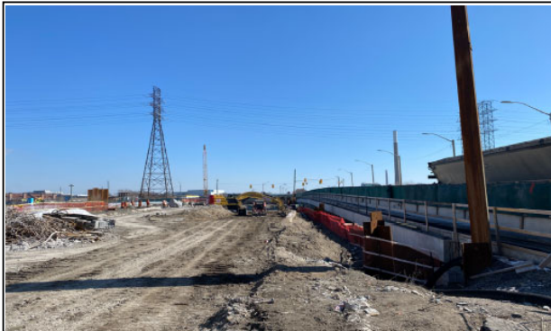
Figure 5 Lakeshore WB Bridge - Lakeshore WB Bridge Construction
