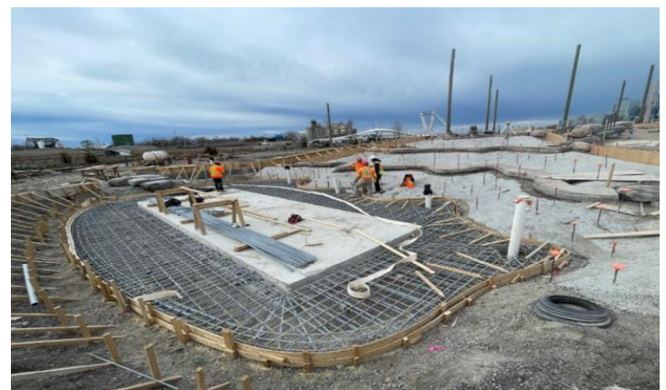
Figure 6 River Park North (Badland 3) - Shotcrete forming & Rebar Installation & Stonework
