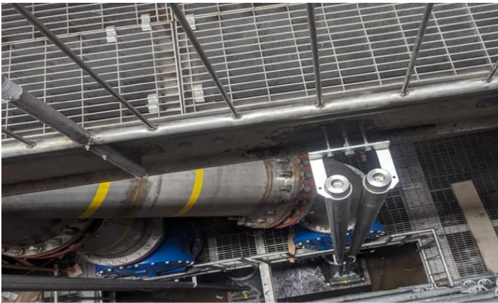
Figure 3 Storm Water Treatment Facility - Electrical Work
