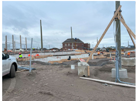
Parks – Playground works ongoing ;
