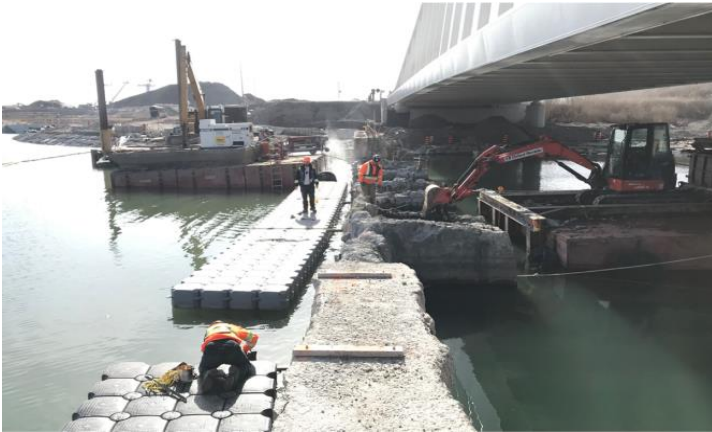
Figure 1 West Plug - Removal of Diaphragm Wall
