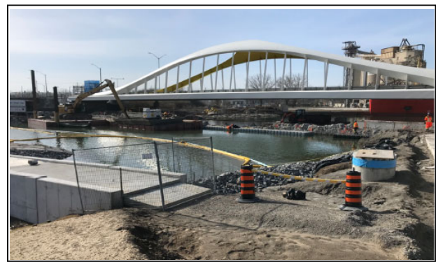
Figure 2 West Plug- Removal of Diaphragm Wall
