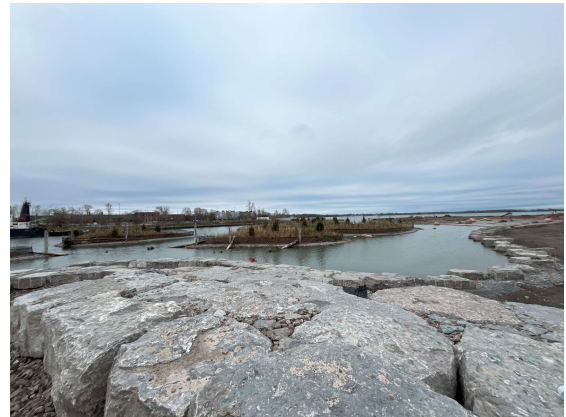
Canoe Cove – Armour stone placement;
