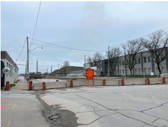
Villiers St. – road works in progress;
