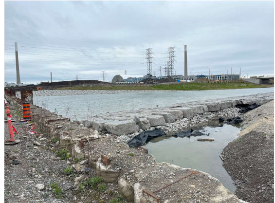
River Channel – River flooded, excavation near the north plug area is ongoing;
