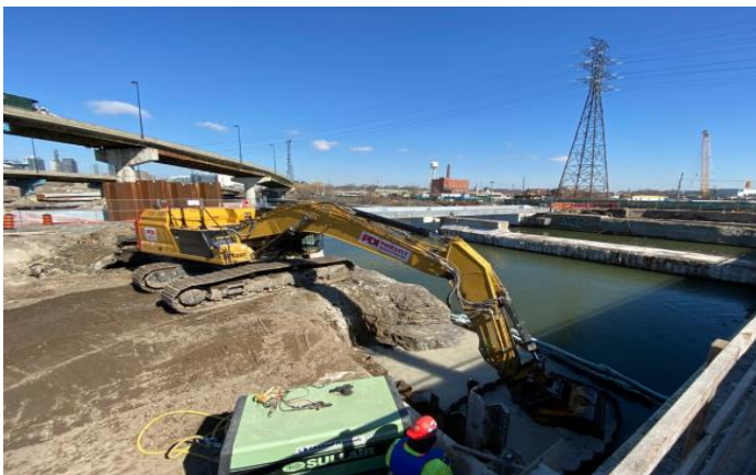
Figure 5 Lake Shore Westbound Bridge - Removal works at Bent 334
