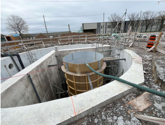
Villiers Road – Utilities Shaft work in progress;
