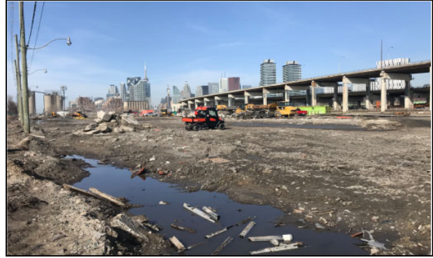
Figure 4 Villiers Underground Utility Removal
