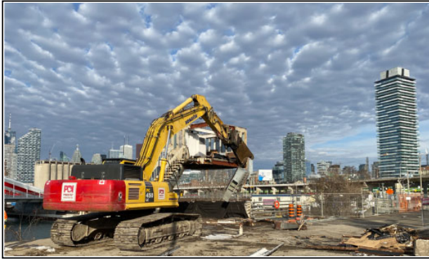
Figure 3 Old Cherry Bridge Demo - Removal of Operators Booth
