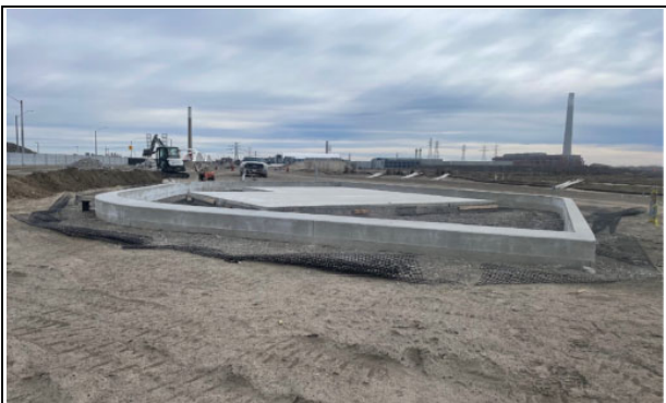
Figure 7 River Park North- Reaching Racoon- Concrete Foundation and Curb
