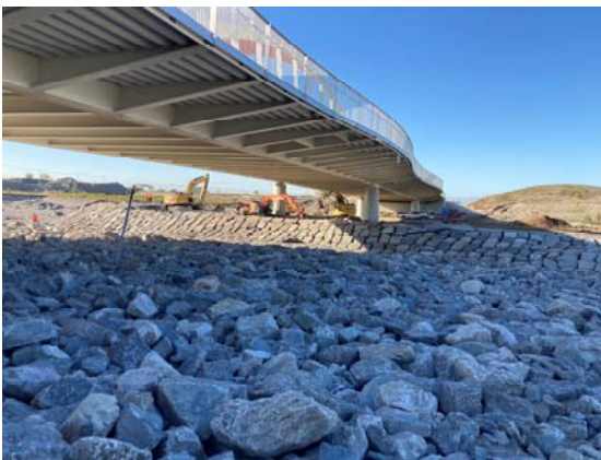
Commissioners Bridge – Stone filling gaps in progress;
