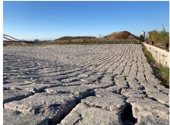
River Channel – Armour stone installed, filling gaps with smaller stones ongoing;
