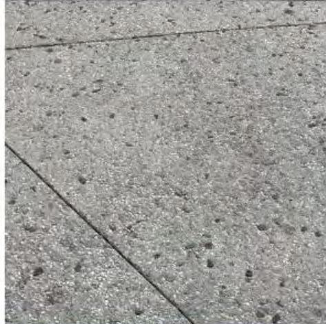
Exposed Aggregate Concrete with granite aggregate and special saw cuts
