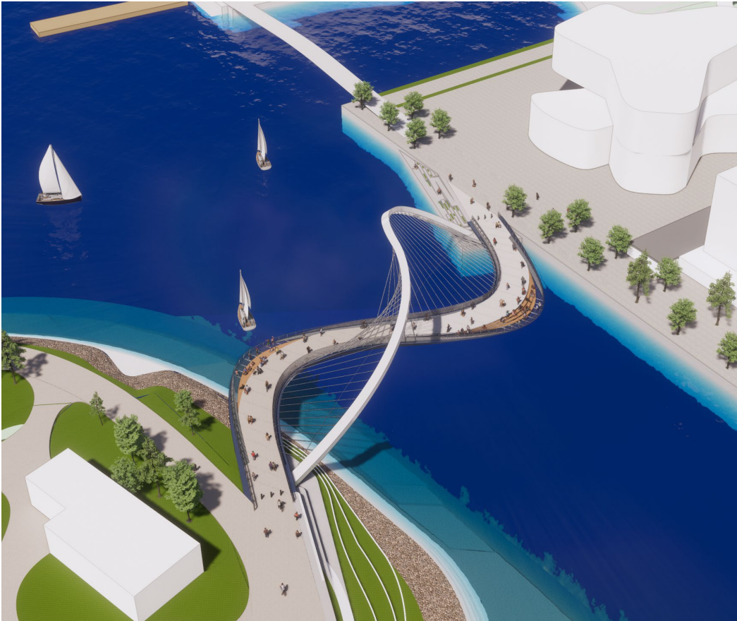
Bridge Deck Geometry and Anti-funicular Arch selected for development in final design
