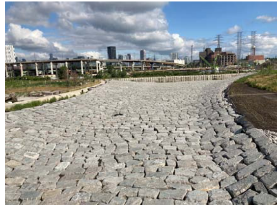
River Channel – Armour stone installed;
