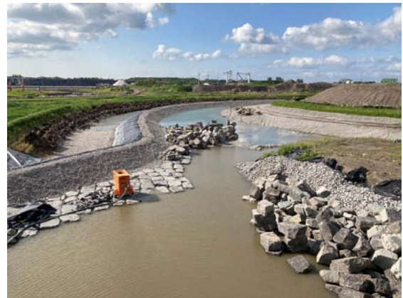
New River and River Valley – Armor stone in edges in place, river valley planting in progress;
