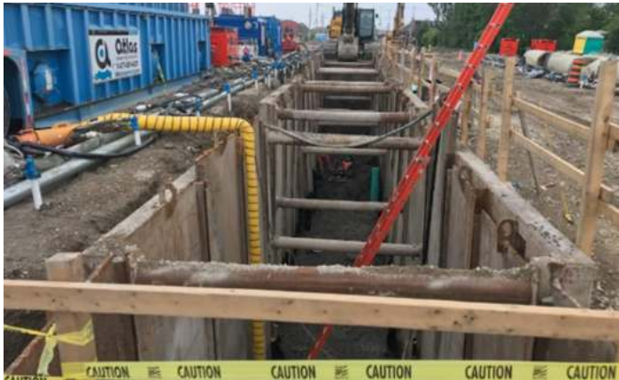
Figure 3 Wet Utility Installation at Commissioner Street
