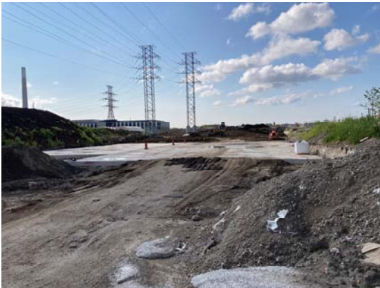
New Don Roadway – Bearing concrete slab poured;
