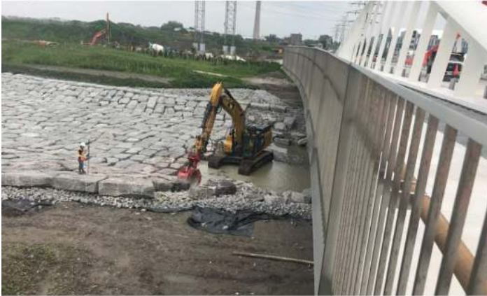
Figure 1 Armour stone placement at River Channel
