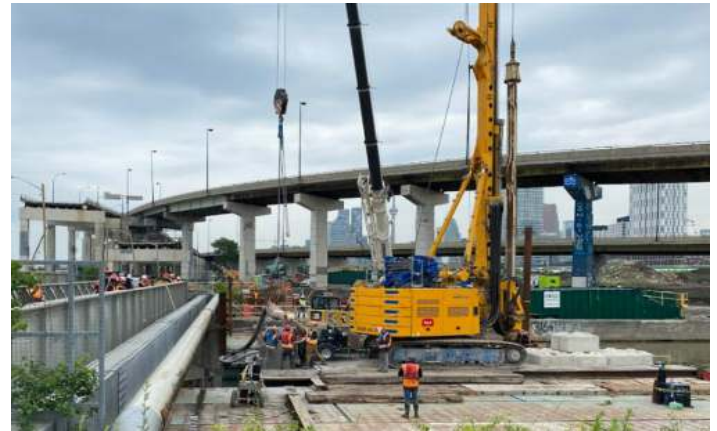
Figure 4 Installation of Micropiles at Lake Shore Utility Bridge
