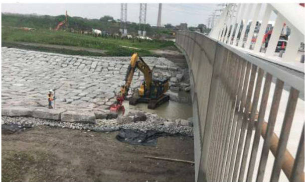
Figure 1 Armour stone placement at River Channel
