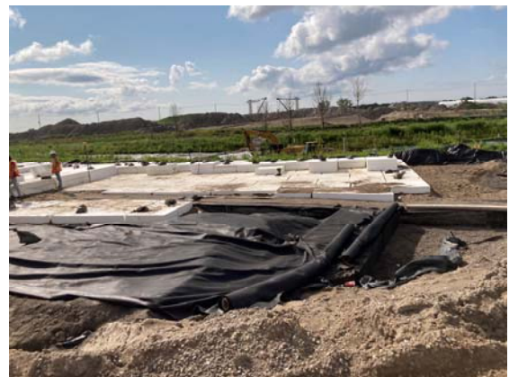
River Vally – Styrofoam installation to help with sagging works in progress;
