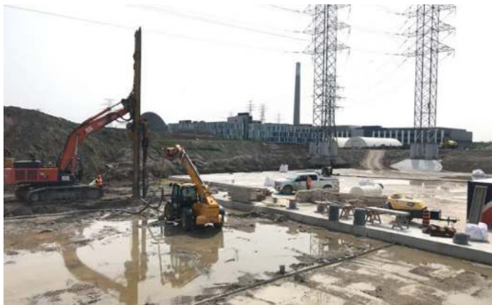
Figure 5 Rigid Inclusion and Load Transfer Platform at Don Roadway South
