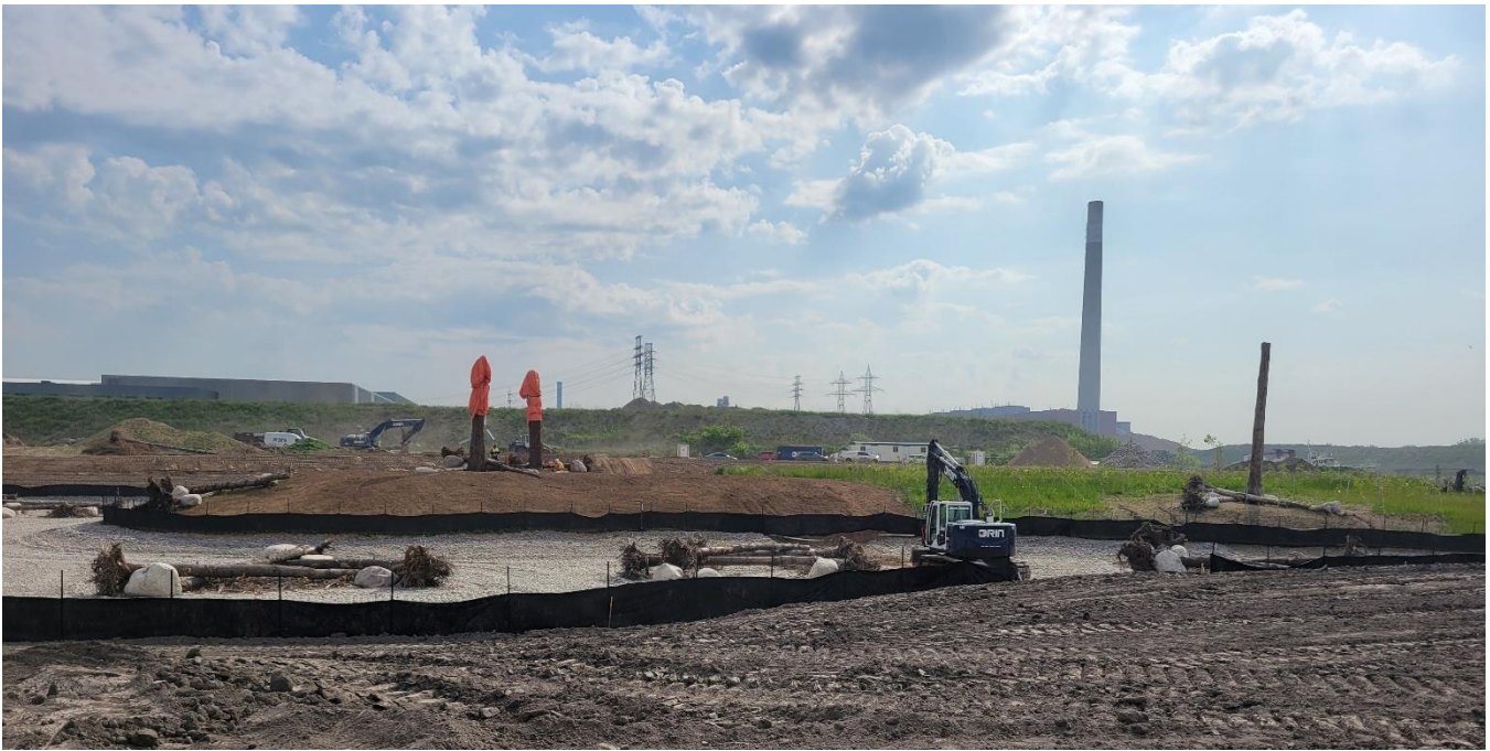
Above: The tree trunks covered in orange tarp have been installed as habitat for chimney swifts in the Don Greenway. The tarp is there because we aren't quite ready for them to move in yet.
