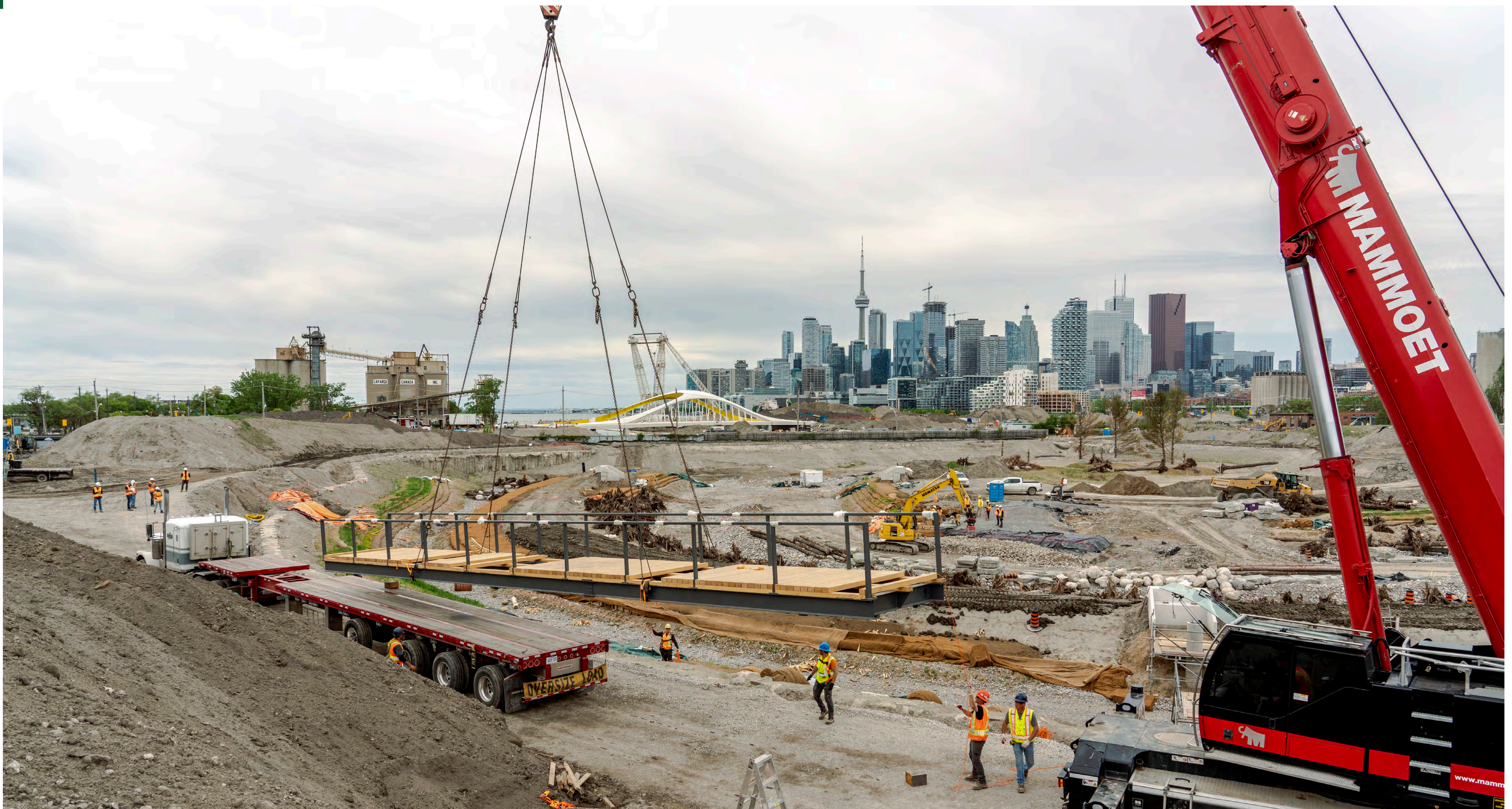
Looking west over the river valley under construction as crews place a new pedestrian bridge. In the distance, one of four new bridges connects people travelling along a newly aligned Cherry Street.
