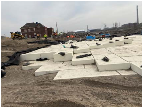
RVPN – Geofoam installation to help with sagging in progress;
