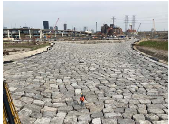
SDMA at River Channel – Armour stone installed;
