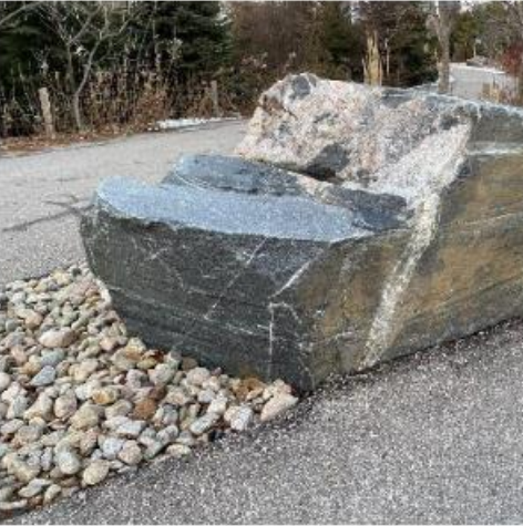
Erratic boulders and River Rock Informal seating edges and stormwater erosion protection
