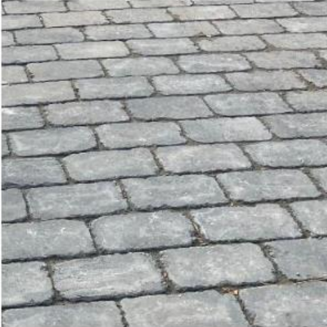
Concrete Unit Pavers Pedestrian Walkway
