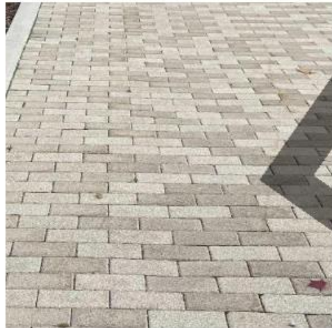
Permeable Unit Pavers Pedestrian Walkway
