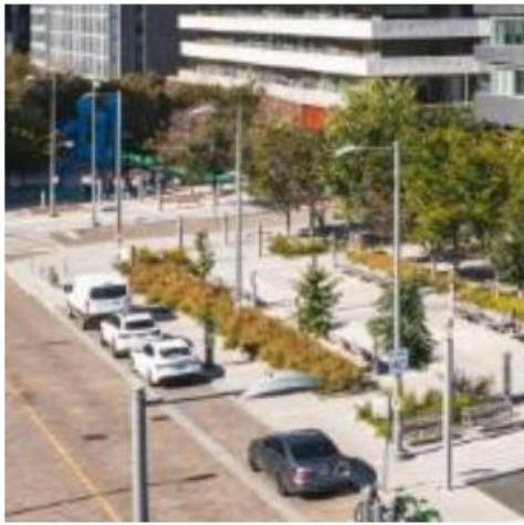
New Waterfront Signature Lighting Aluminium pole with approved new fixture
