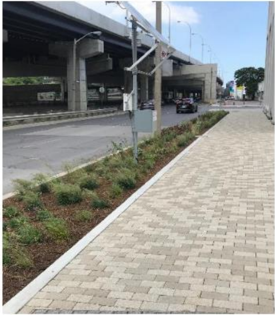
Lakeshore Boulevard East, Green Infrastructure Pilot, 2022
