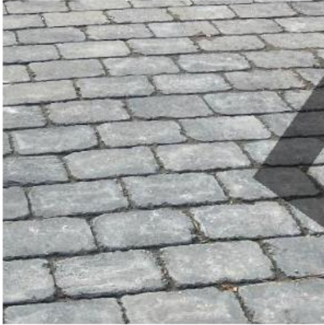
Concrete Unit Pavers Pedestrian Walkway (Building Edges)
