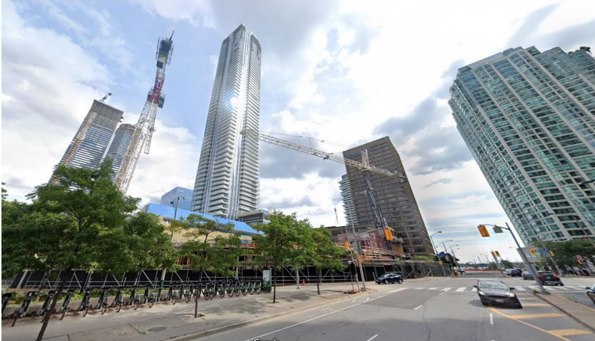
View #1 – Yonge and Lake Shore looking southeast
