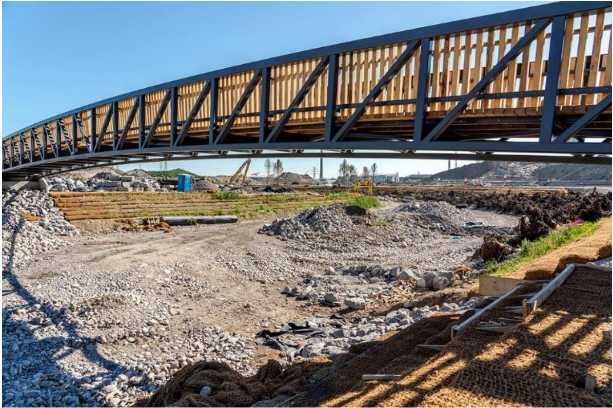
Above: The pedestrian bridge spanning the future river was installed earlier this summer. Under the bridge you can see the river bottom and the river banks in the background.
