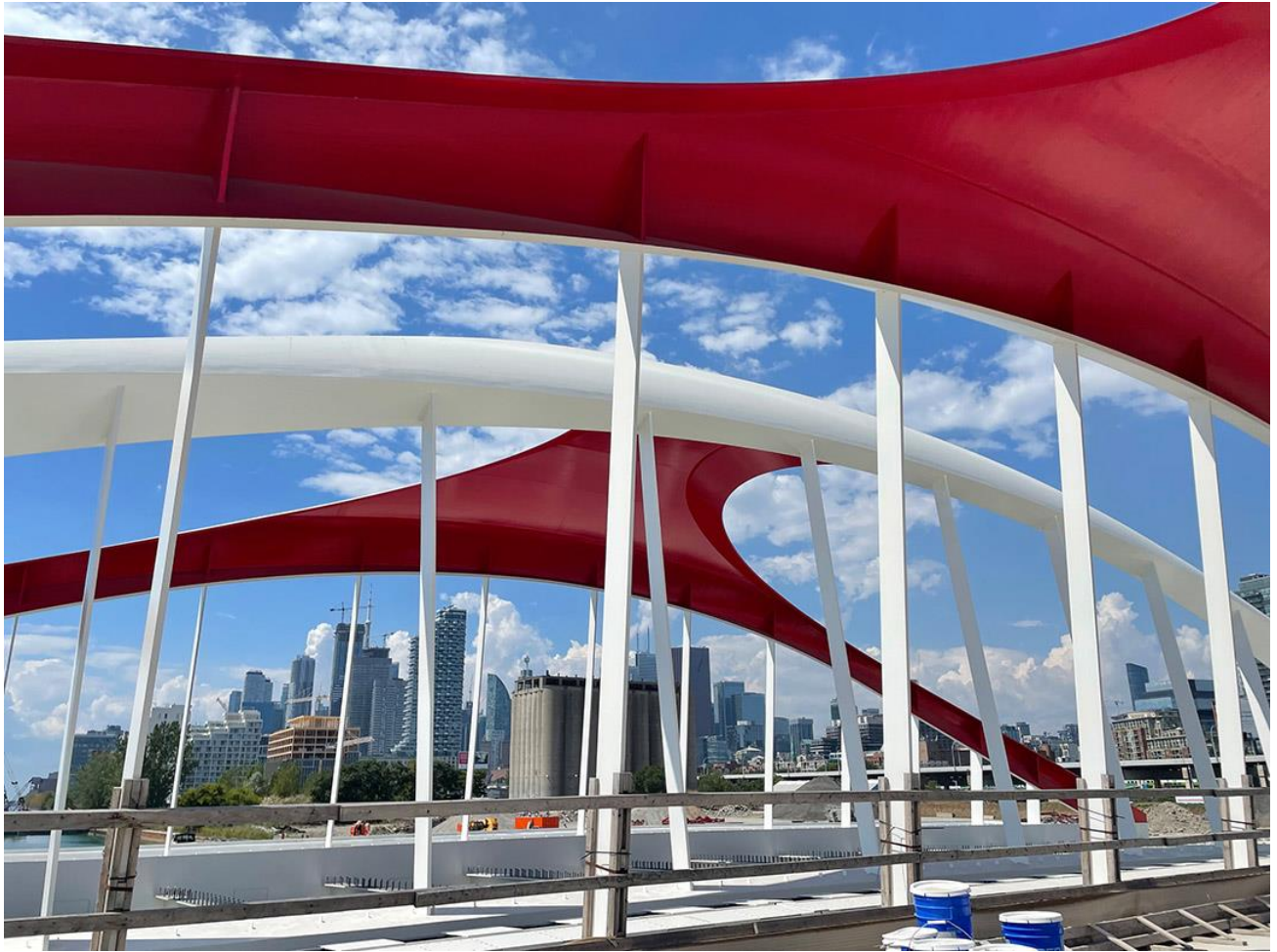
Above: The second bridge for the Cherry Street North crossing arrived earlier this year and has now been installed.
