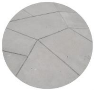
Poured concrete with joint pattern
