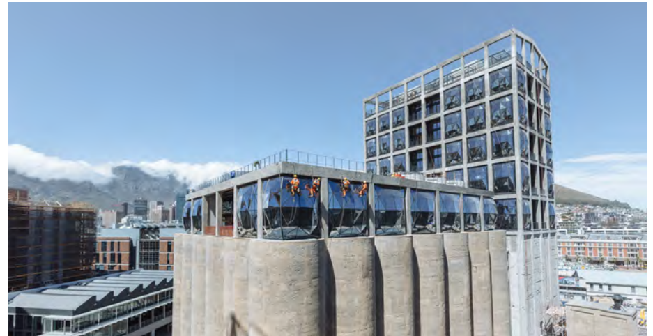
The historic grain silo at the V&A Waterfront in Cape Town, South Africa is being converted into the new home of the Zeitz MOCAA permanent contemporary art collection.
