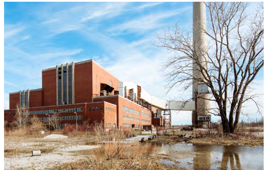
The Hearn Power Station, opened in 1951, was the site of Canada's first 100 MW steam turbo-generator set.
