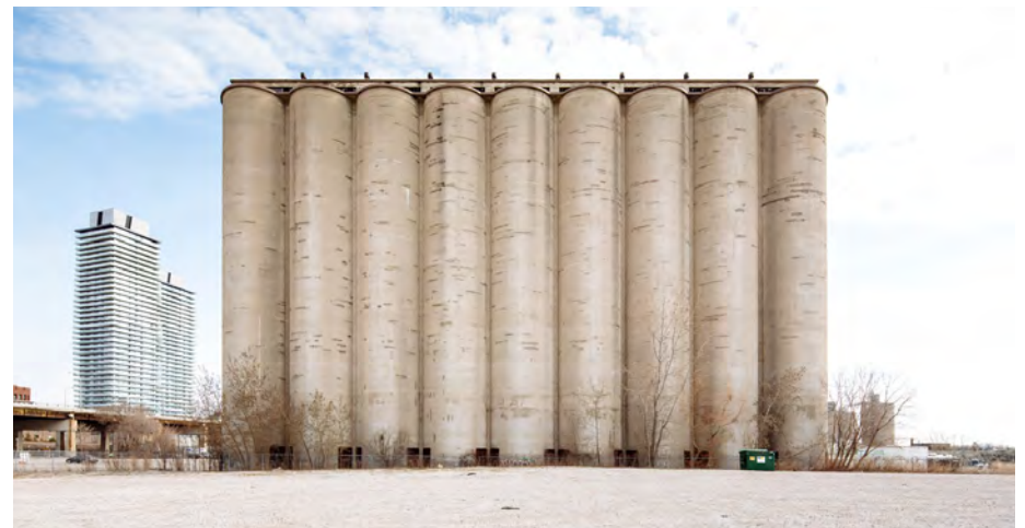
Victory Soya Mills Silo at Quayside
