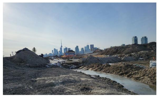
**Above:** Excavation in the river valley is complete. In this photo, you can see a recently excavated section in the foreground. The next step for this section is to complete the installation of the river liner, and then install river finishes.
