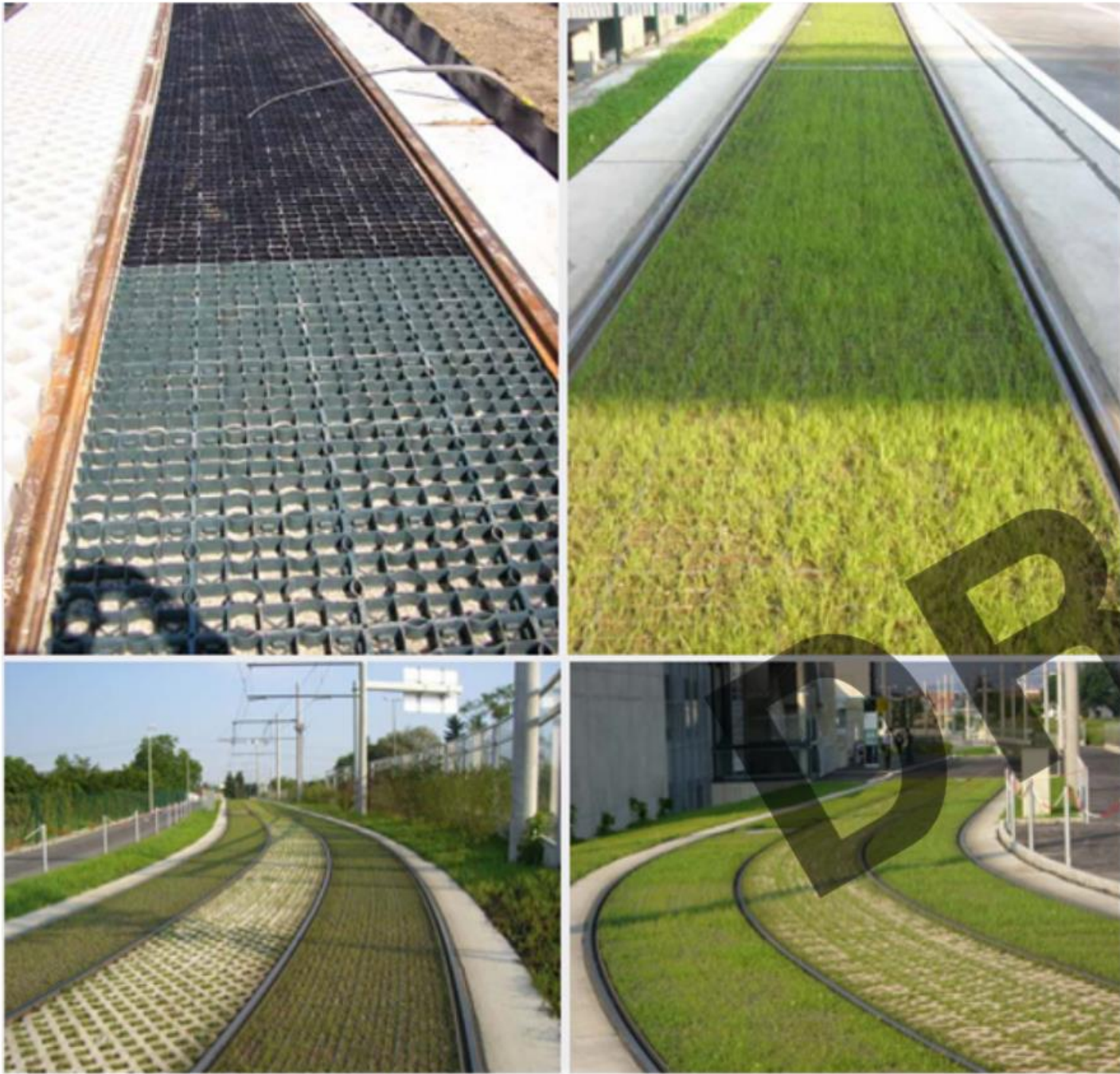
Planted Geogrid System for Fire and Emergency Vehicles Case Study: Graz Liebenau, Austria (2800m 2 )
