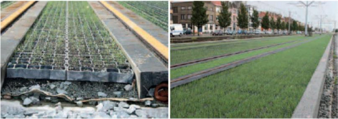
Figure 140: Plastic grass grid system after seeding (Picture: [27])
