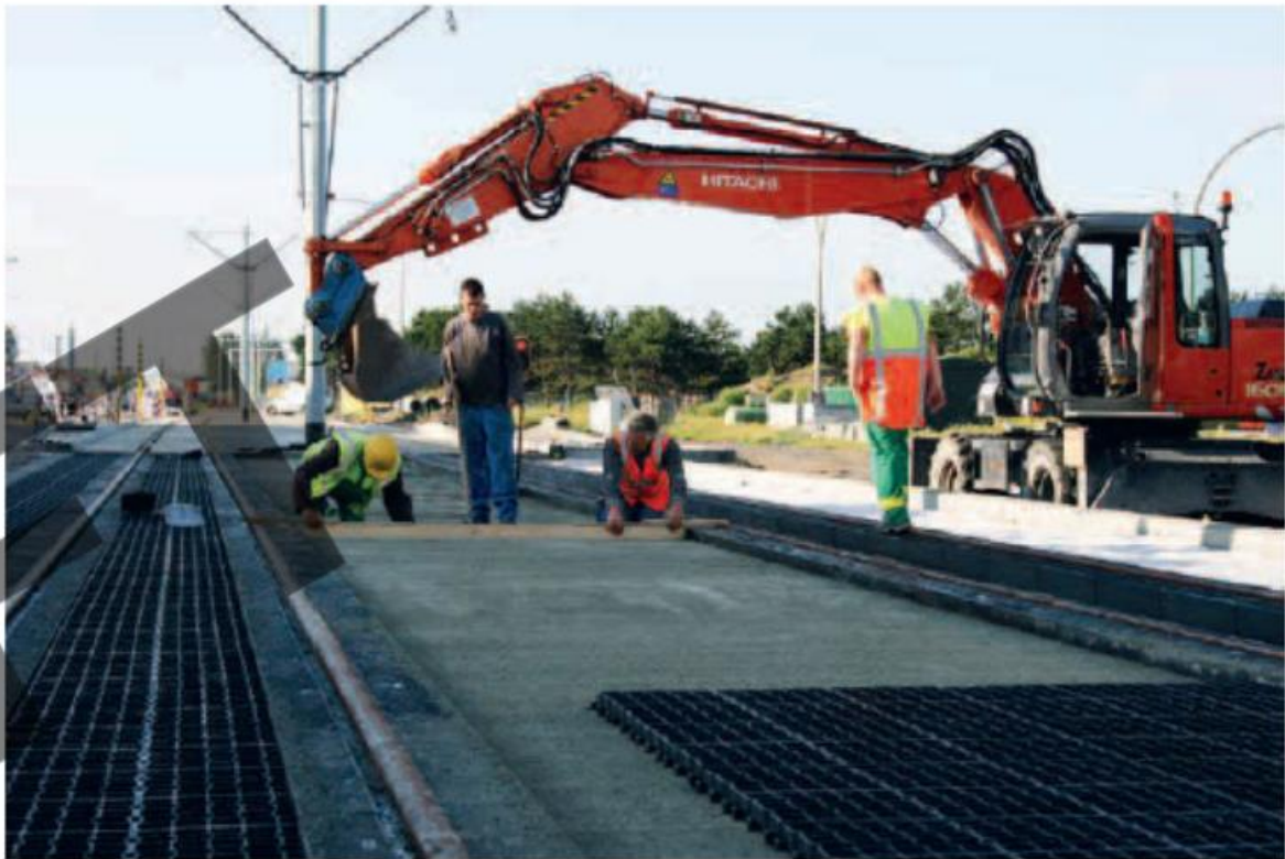
Figure 139: Installation of ECORASTER® plastic grass grid system for seeding of grass (Picture: [27])
