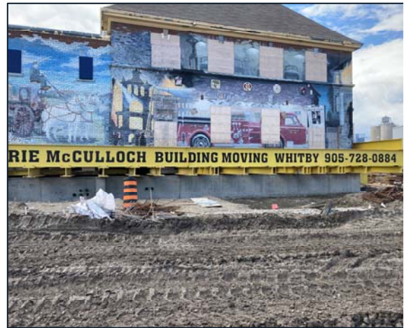
Heritage Building Relocation – Placed onto new foundation inside park boundaries.
