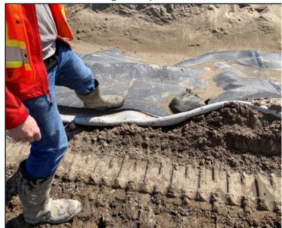
River Valley – Geotextile and membrane installation ongoing.
