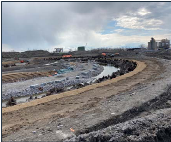
River Valley – Tree Planting and geotextiles for bank protection installation in progress.
