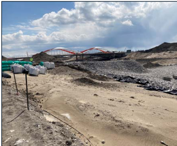
Riverbed at Elbow Area – Stone being placed.
