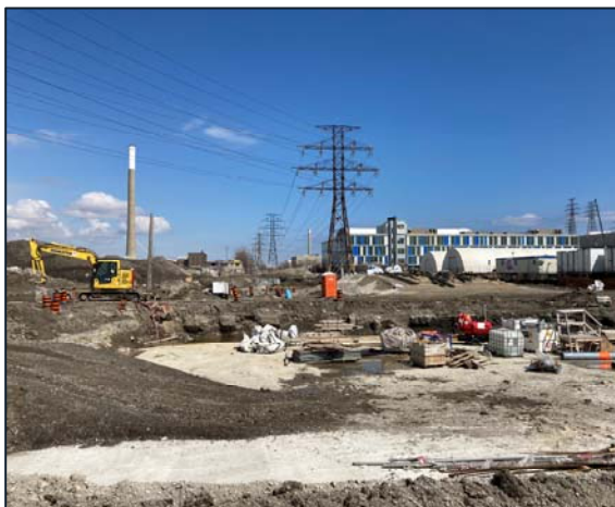
Soil Bearing Capacity Improvement – Structural slab complete.
