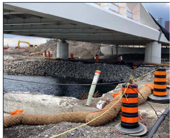
Cherry St. Bridge – In final position on abutments.
