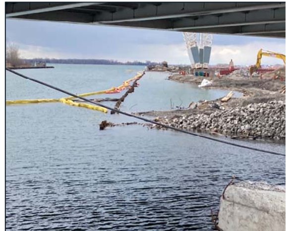
Polson Slip – Backfill and shore alignment in progress.
