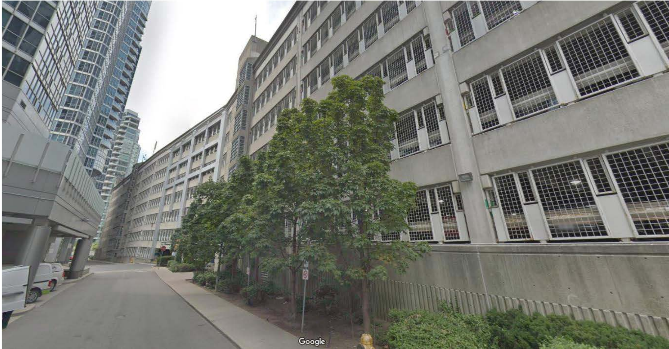
South elevation of existing parking structure from the east end of the laneway
