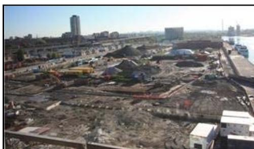
Construction on the south side of Sherbourne Park is making steady progress. Crews began in mid-July by preparing the site and drilling caissons — the deep foundation pillars — required to support the park's pavilion and splash pad/skating rink. Caisson drilling is expected to be complete in August allowing crews to move on to the pavilion's foundation.
