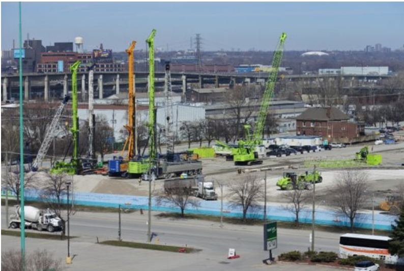
Left: Drill rigs at the construction site east of Cherry Street and south of Commissioners street are ready to start installing secant piles along the shoreline of the new river valley as we begin deeper excavation.
